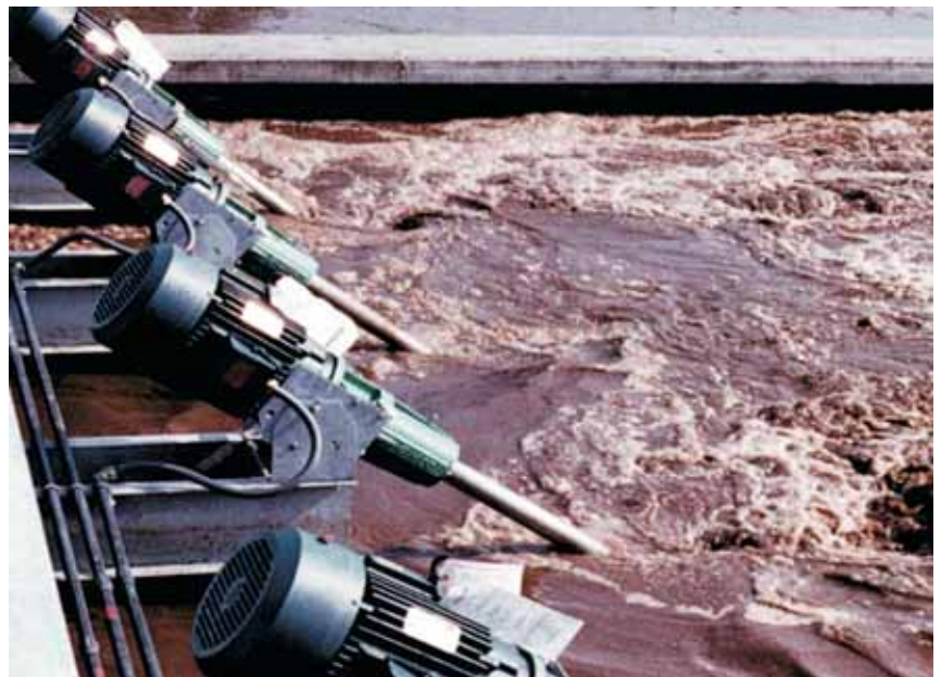
(Photo Right) Fixed, bridge-mounted units in an oxidation ditch.
