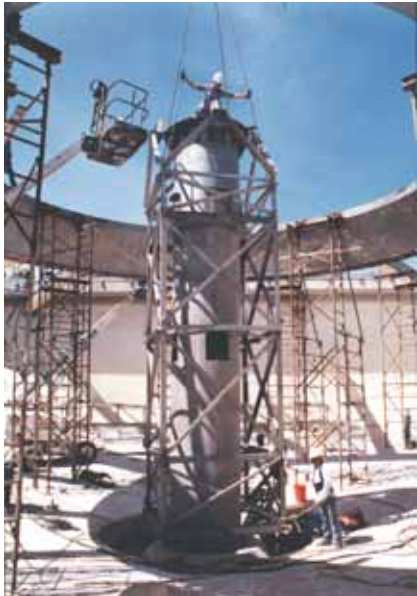
Type HRC Reactor Clarifier, showing installation of torque case over center column
